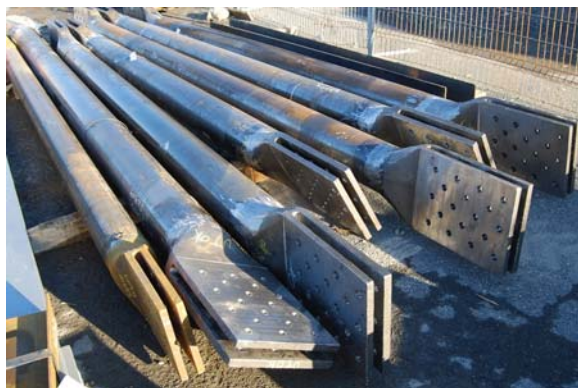
Figure 9: Braces equipped with Cast ConneX™ High-Strength Connectors on site awaiting installation (left); braces installed in the steel frame structure (right)
