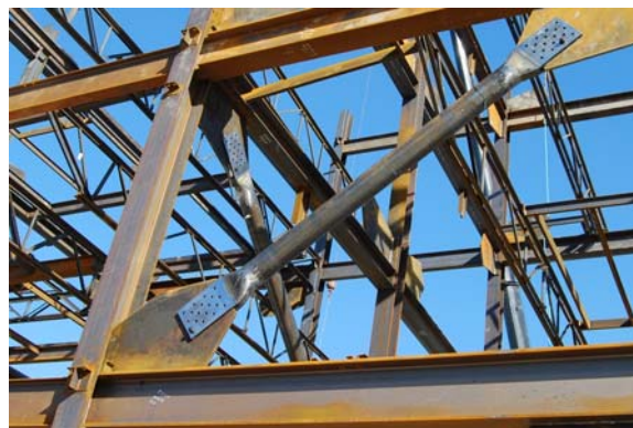
Figure 9: Braces equipped with Cast ConneX™ High-Strength Connectors on site awaiting installation (left); braces installed in the steel frame structure (right)
