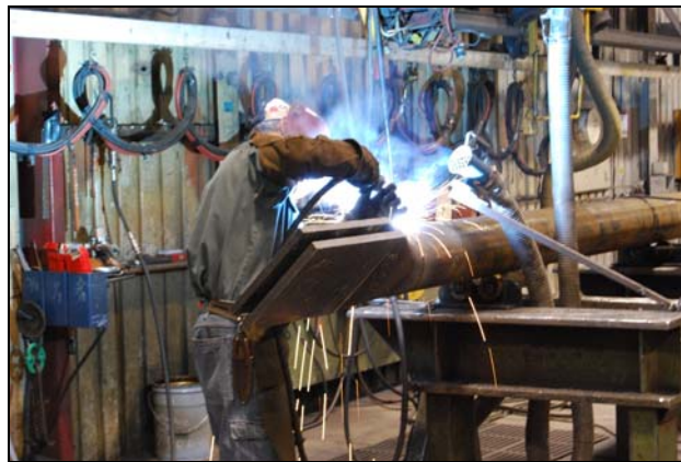
Caption: Canam Group welder securing a Cast ConneX™ High-Strength Connector to a round hollow structural section brace member for the Sandoz project.
