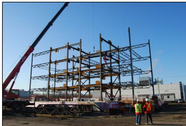
Caption: Sandoz Canada Administration Building during construction.
